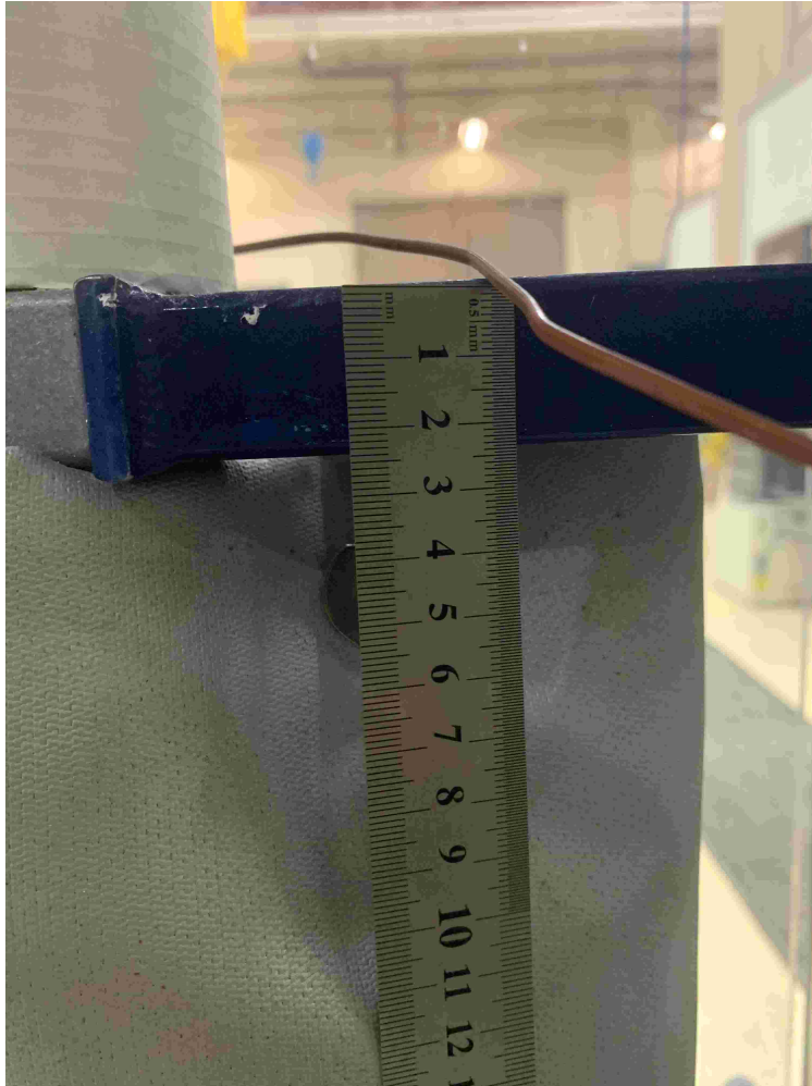
Figure 2.28: Photograph of showing Support Structure Width of about 2.3 to 2.4 cm in CIET near DHX Branch, Credit Omar Ashraf Alzaabi
