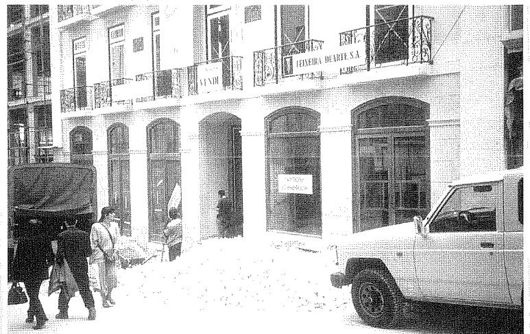
New shop facades in a reconstructed building on Rua Garrett, with courtyard entrance in center.
