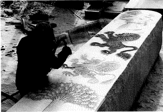
A master sand blaster creating one of the obelisks for the Radnor Gateways Enhancement Project.
