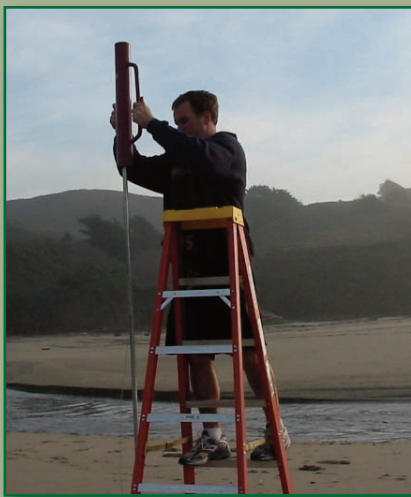
Stanford graduate student Nick de Sieyes installs a monitoring well at a Northern California beach.
