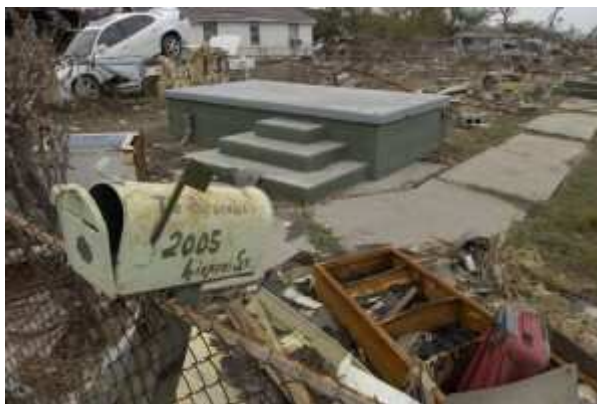
Image 6: This mailbox was all that remained of a home in New Orleans's Lower Ninth Ward. 287
