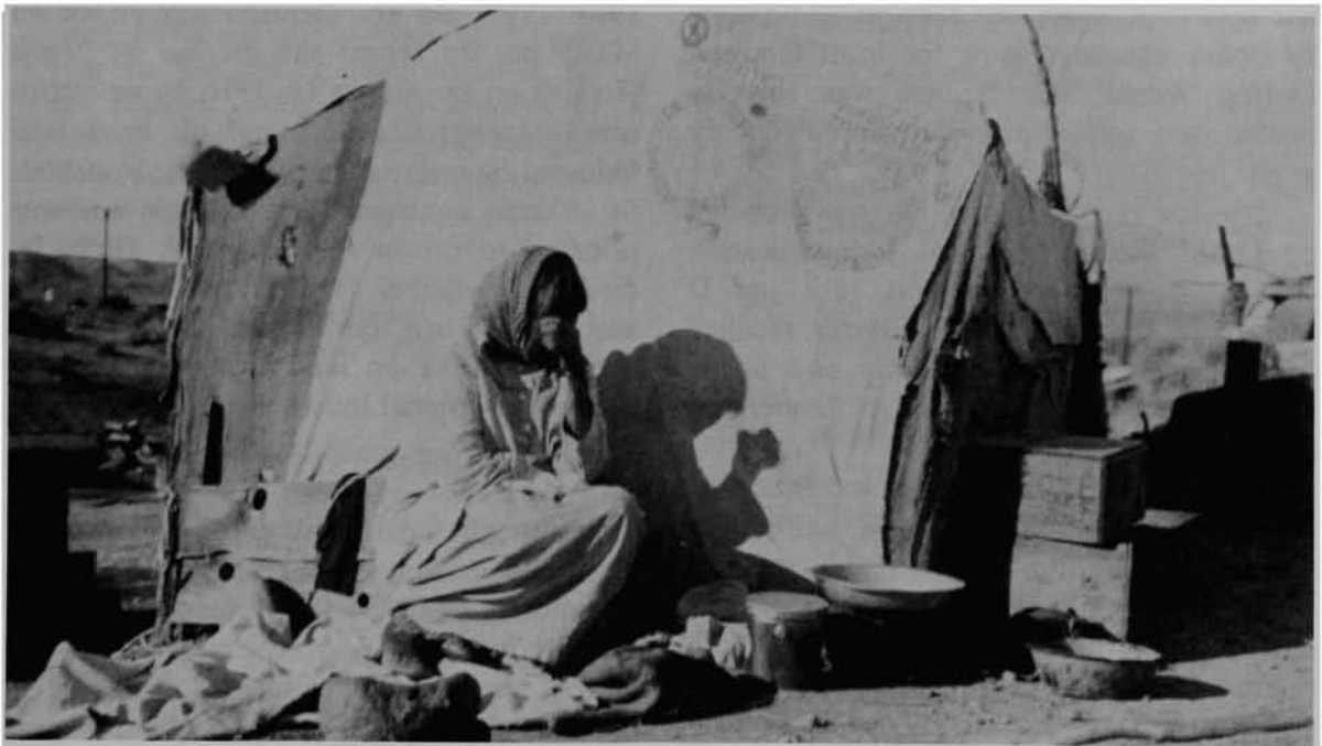
Fig. 4. "Old Susie Feb. 5, 1923." Close-up of Susie Higgins seated in front of her house in Victorville. Exterior of hut is covered with discarded cloth cement sacks from the Southwestern Portland Cement Company established in Victorville in 1917. Photo courtesy of Jean Durfee.
