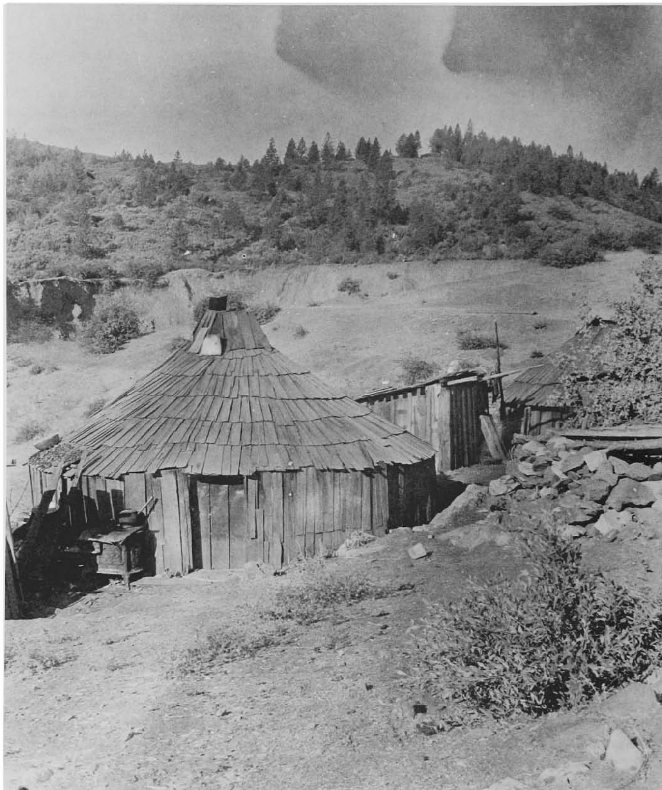
Fig. 10. Yellowjacket's conical house and shack, 1900 (courtesy of the Bancroft Library, University of California, Berkeley).
