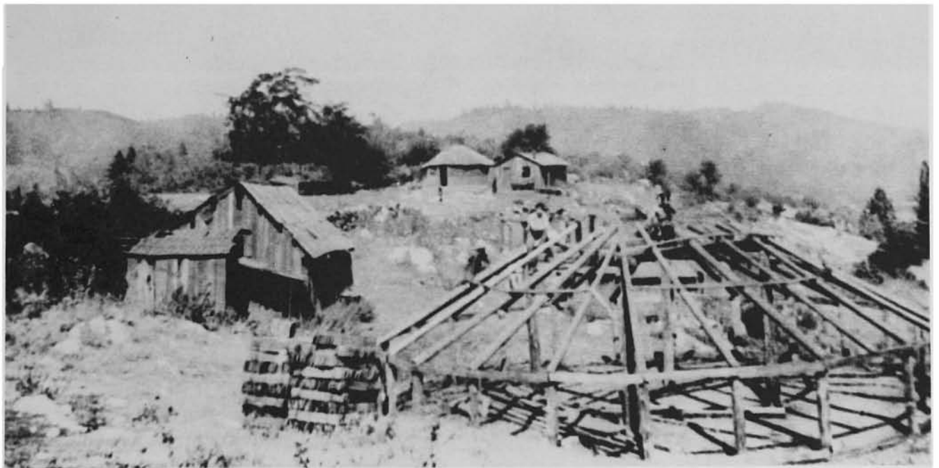
Fig. 8. Murphys Rancheria. Ceremonial Roundhouse under construction, 1901 (courtesy of Milton B. Smith).
