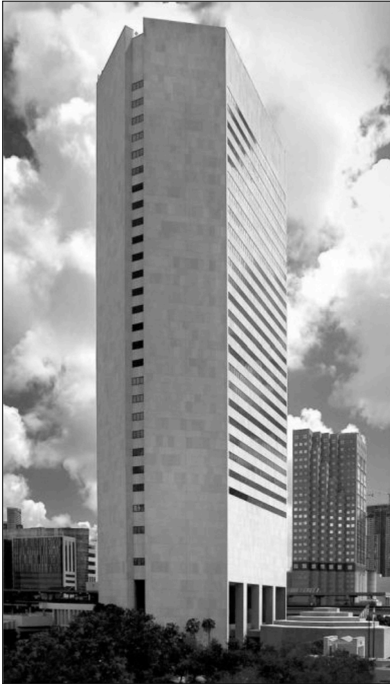
Figure 5 Stephen P. Clark Center. Source: http://www.danlepore.com/case-studies/stone-construction/miami-dade-centerstephen-p-clark-government-center
