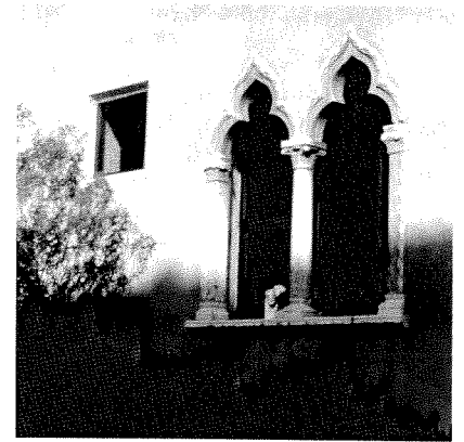
4 Scarpa backed the Gothic windows, added during a 1920s renovation, with modern windows.
