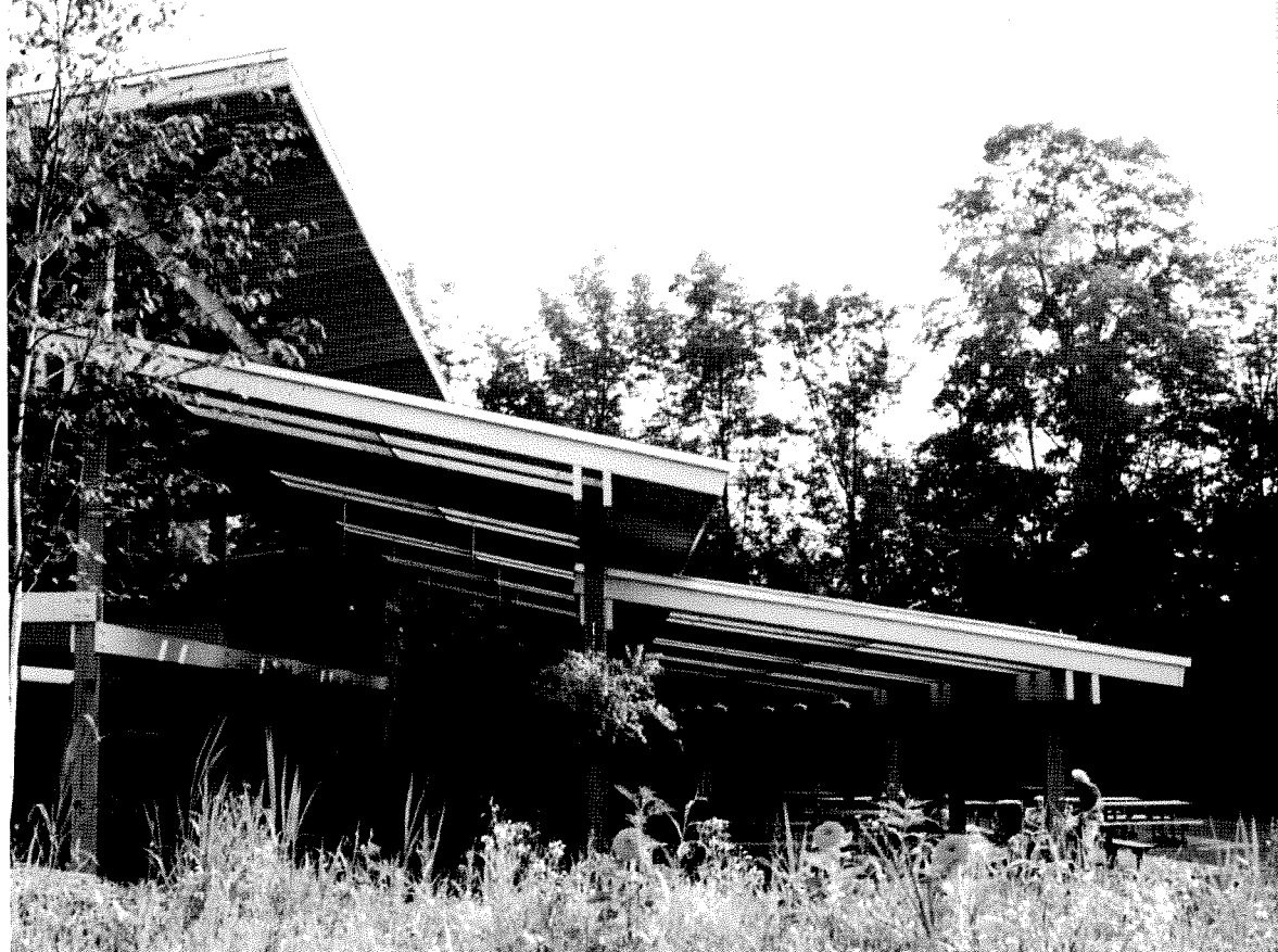
above: The Music Shed restroom building incorporates both ventilating clerestory awning windows and fixed clerestory glazing. Rafters and trusses are left exposed.
