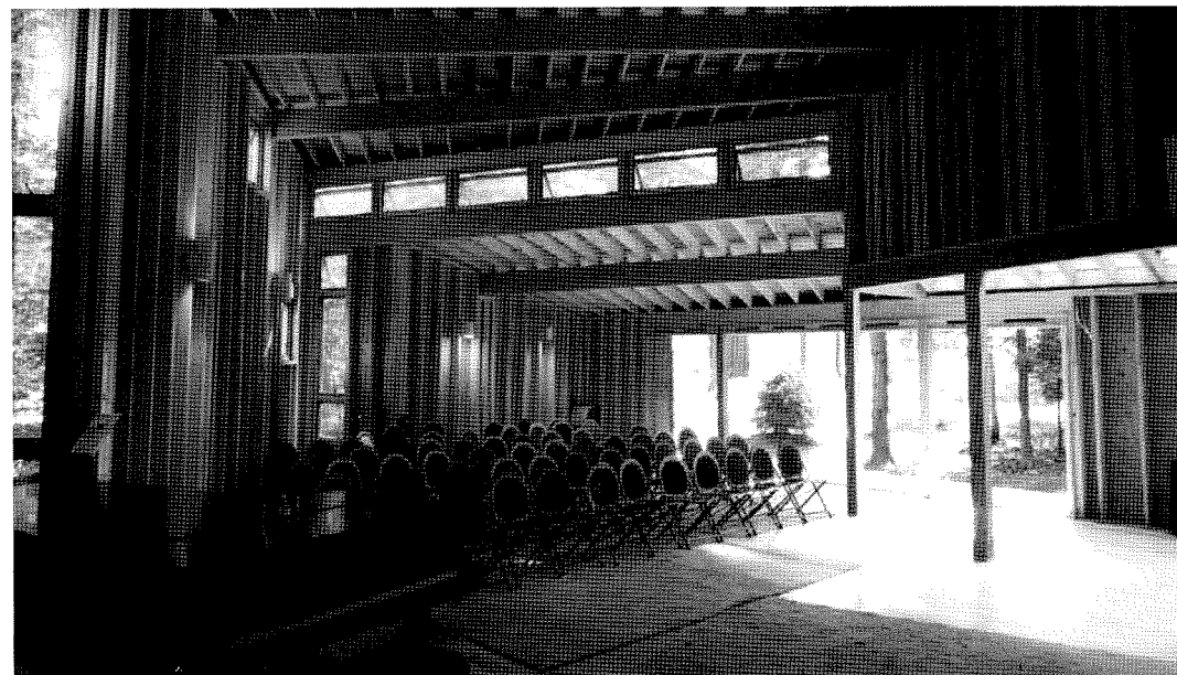
right: Clerestory and high vertical windows offer natural ventilation for the Rehearsal Hall. Studs, beams and rafters are exposed, providing acoustics that are well suited for soloists and for small and large ensembles. The sliding doors are open and face the Performance Path.
