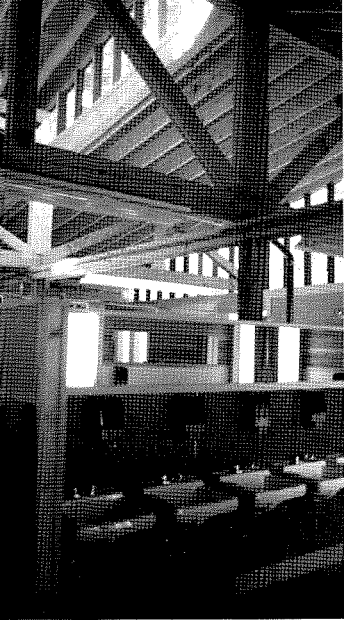
above: The Music Shed restroom building incorporates both ventilating clerestory awning windows and fixed clerestory glazing. Rafters and trusses are left exposed.
