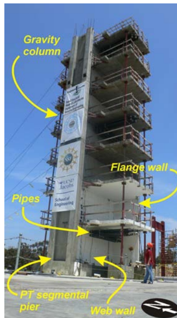
Figure 7.1 South West View of Building.
