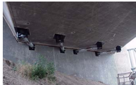
(c) Viscous fluid damper used on 91/5 Overcrossing
