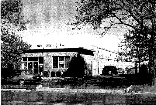
Above: Typical suburban industrial building, with articulated front office.
