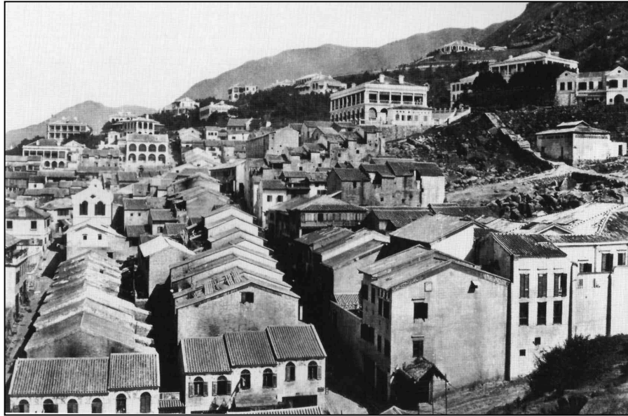
Figure 13: Photo of Central and Sheung Wan districts (also referred to as the Tai Ping Shan district) c1868. The photo depicts colonial-style buildings sitting atop a hill looking down upon Chinese-style buildings (Photo from Bremner and Lung 2003).
